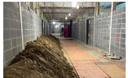
Above: First floor corridor excavation for plumbing
